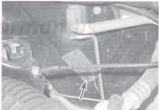
Safety compliance plate location (arrow)
